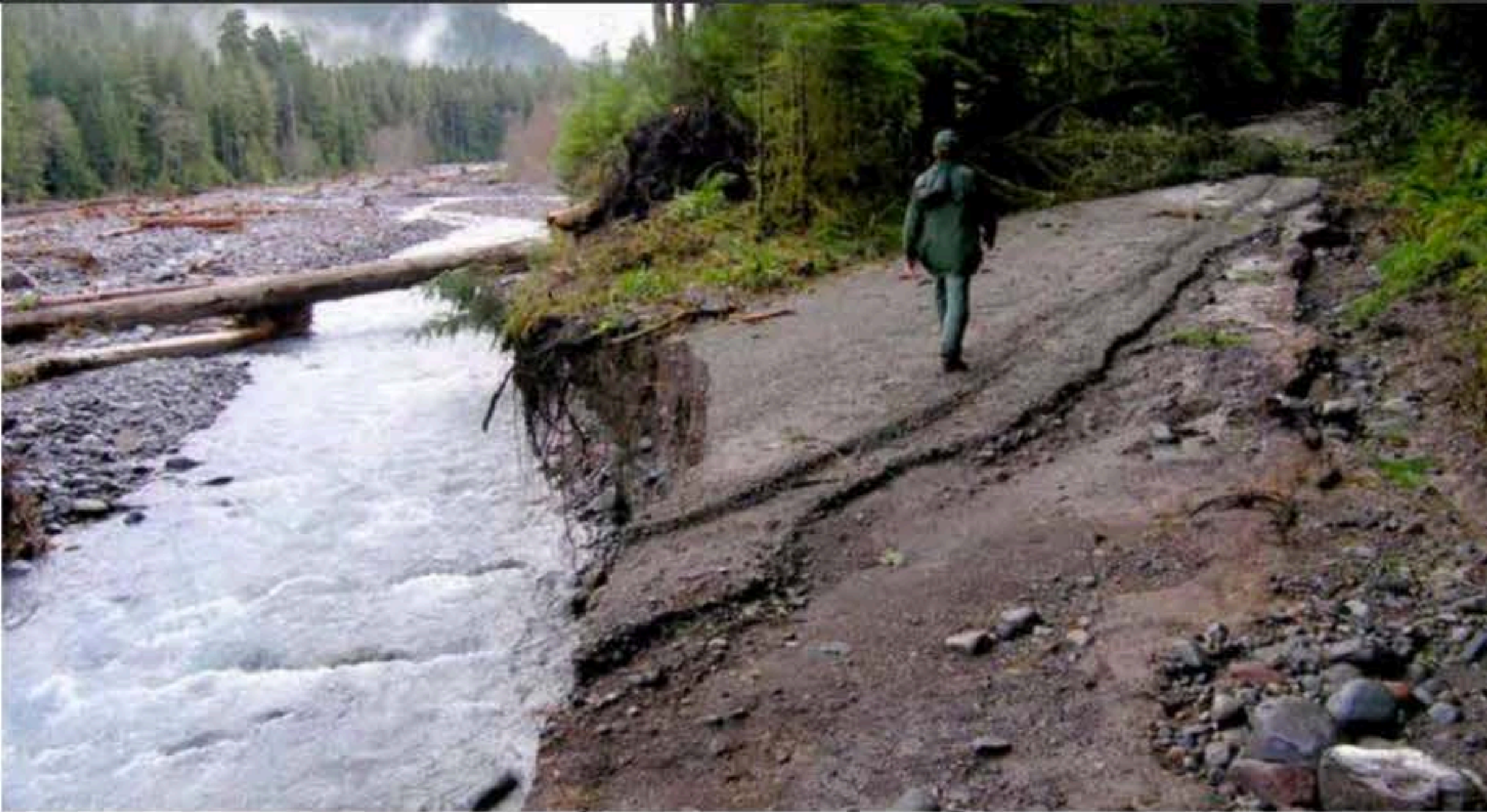
KRISTINA HILL The Carbon River Road in Mt. Rainier National Park washed out in 2006 from flooding that has become more frequent as Rainier’s glaciers melt and carry more sediment into the river channel, causing it to overflow—sometimes right onto the road bed itself, literally turning the Carbon River Road into the Carbon River. This is an important image because it shows the permanently closed road as a ruin that only hikers can access. When I look at this image, it reminds me that climate change will bring an aesthetic of ruins, of poignancy, of loss that some may find romantic, or sublime, or painfully sad. How will designers respond to the proliferation of ruins, of Carbon River Roads?
